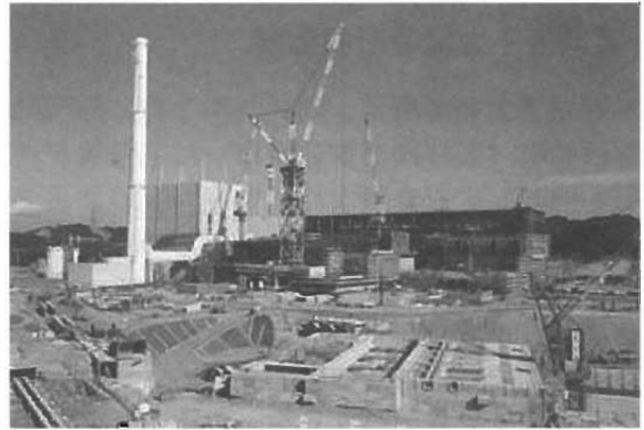
Fig.7 Unit 2 Under Construction(this side)
