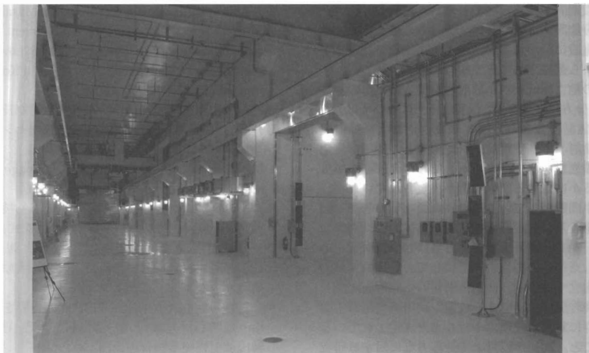
Photo 2 Ground Support Facility (under construction)-Waste Inspections Section
